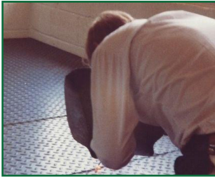
1980. Mr Jenkinson welding the brewing platform, still in use today.
